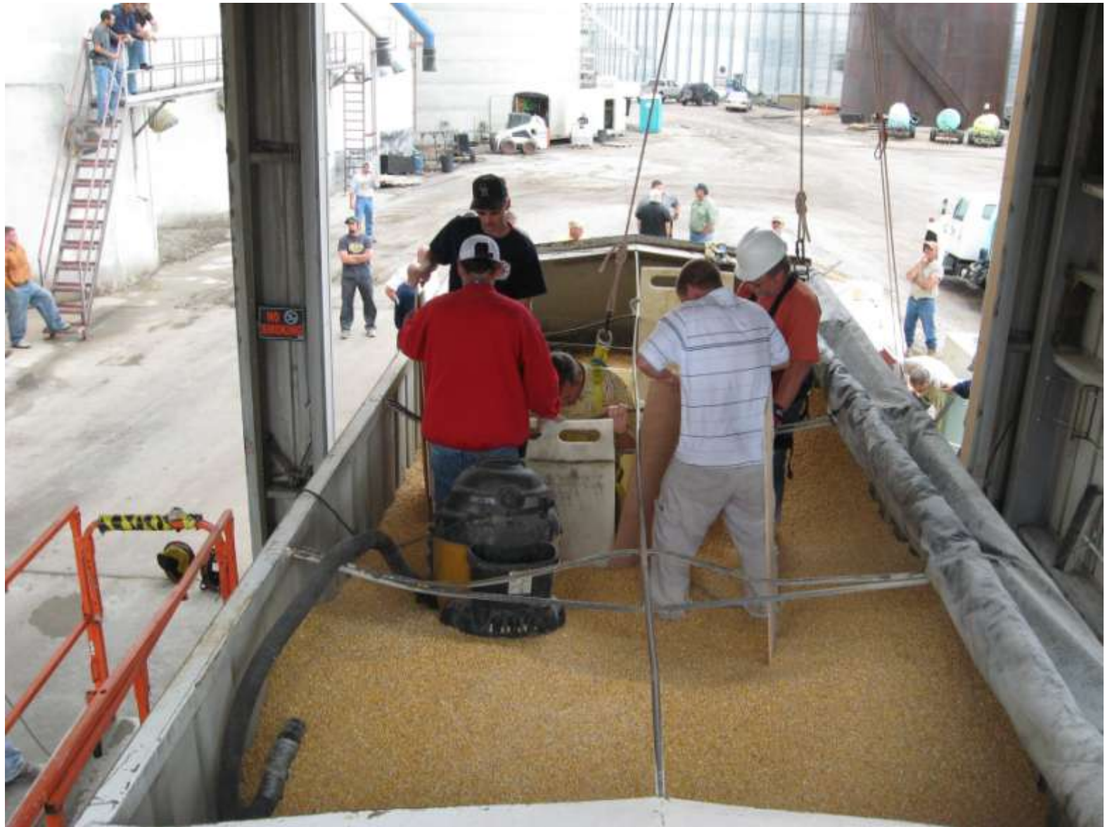
Cofferdam being put in place.
